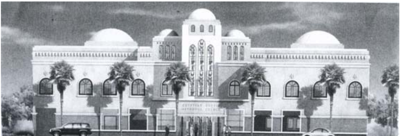
The Great St. Mina's Church for the Coptic Orthodox in Dubai
